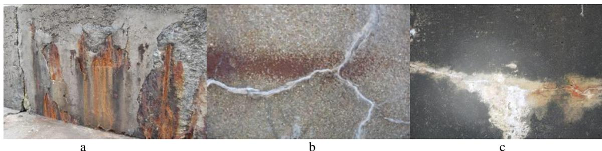
**Figure 4.** The marine environment corrosion on the reinforced concrete of the dams located along the beaches on 2 Mai (a), Neptun (b), Costineşti (c).
