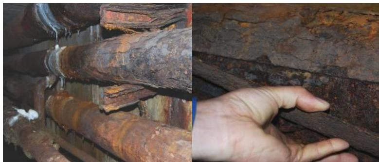
**Figure 2.** The corrosion appearances of the metallic elements caused by marine environment, the Hydrotechnics Node Năvodari.
