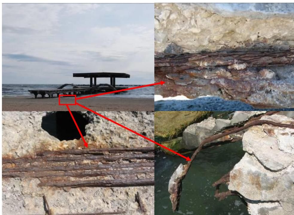
**Figure 3.** Reinforced concrete bridge, carried out in 1935, Mamaia. Different affected sections by the seawater corrosion were present.
