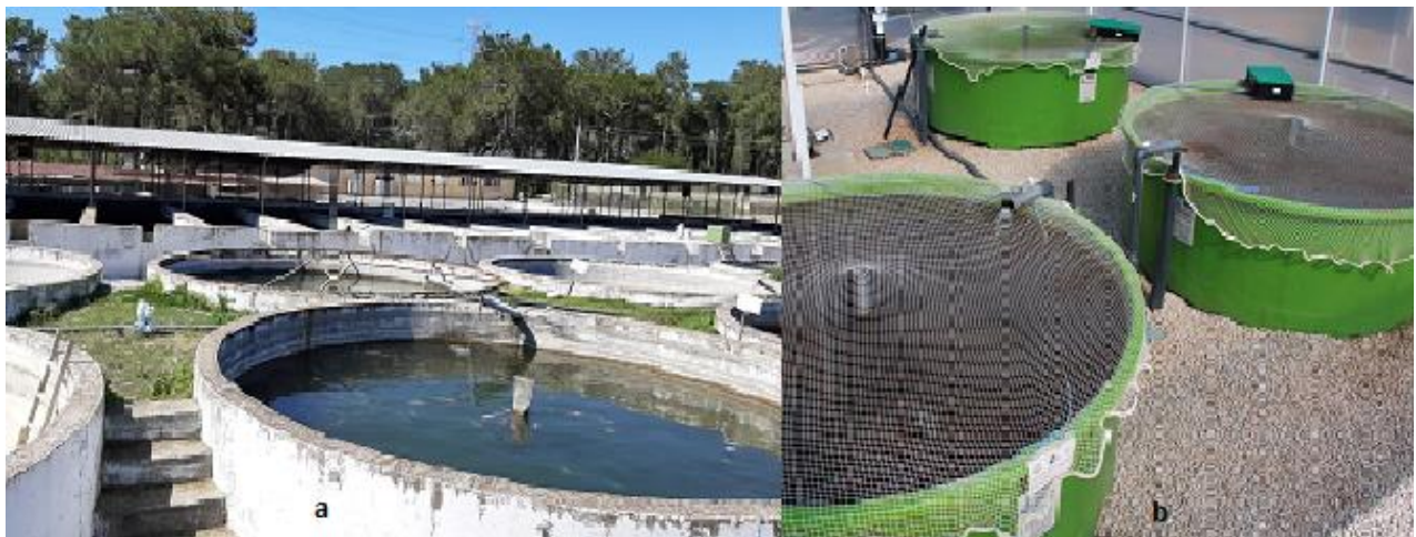
Figure 1. a) Picture of a concrete tank, b) Picture of a fiberglass tank
