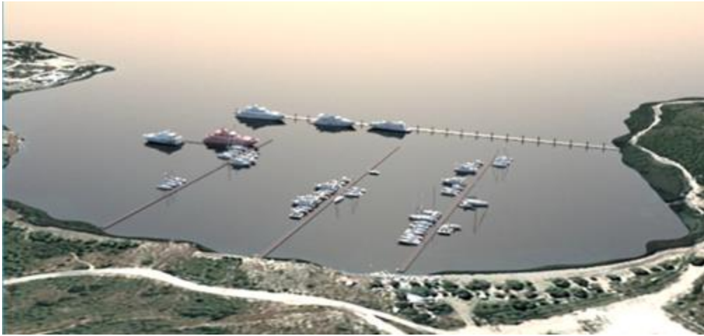
Figure 5. An example of the Floating Berthing and Mooring Facilities.
