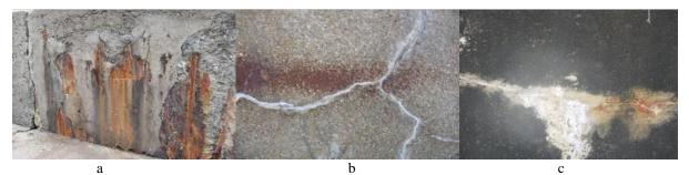
**Figure 4**. The marine environment corrosion on the reinforced concrete of the dams located along the beaches on 2 Mai (a), Neptun (b), Costinești (c).
